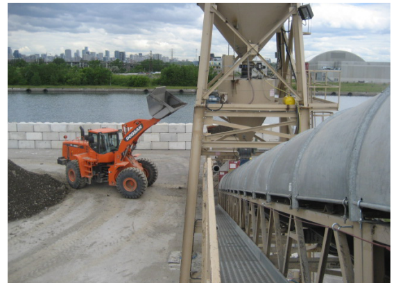
Figure 2. Site using in-situ cement stabilization of contaminated soils.
