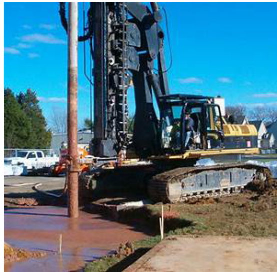
Figure 3. Ex-situ mixing of cement with contaminated soils.
