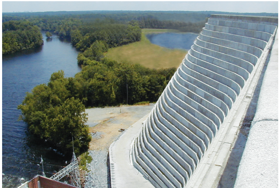
Lake Murray Dam Project in South Carolina
