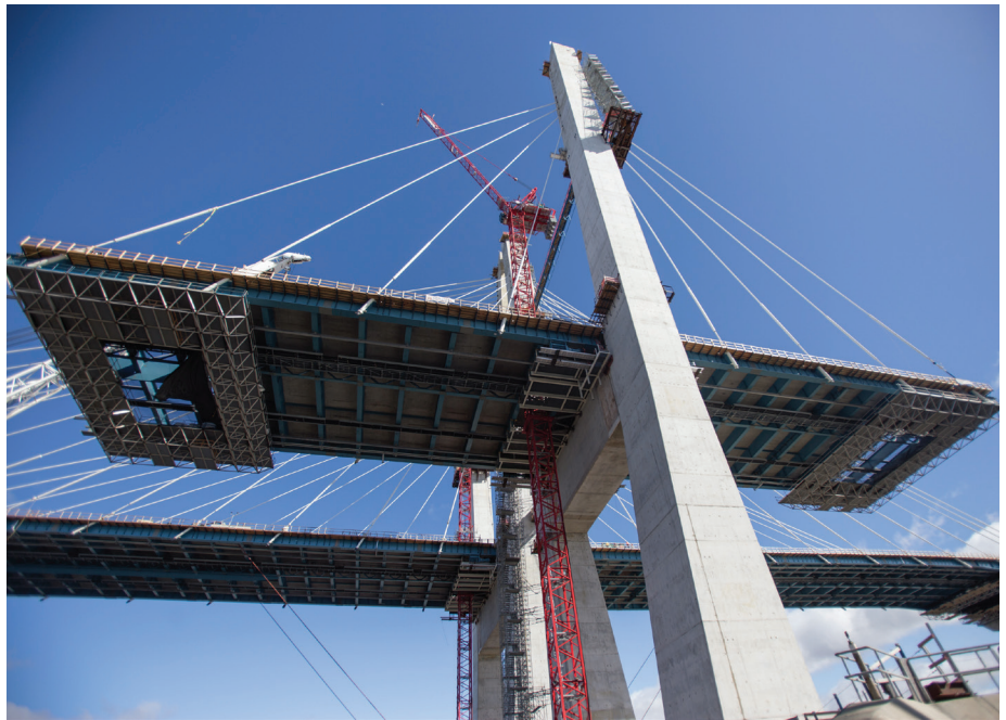
NewCem® Slag Cement – Tappan Zee Bridge
