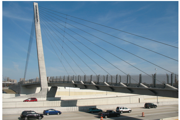
Detroit-Mexicantown Bagley Street Pedestrian Bridge
