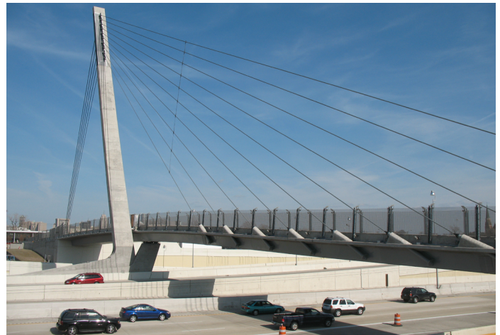
Detroit-Mexicantown Bagley Street Pedestrian Bridge
